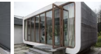
A prototype of Dubai office buildings
